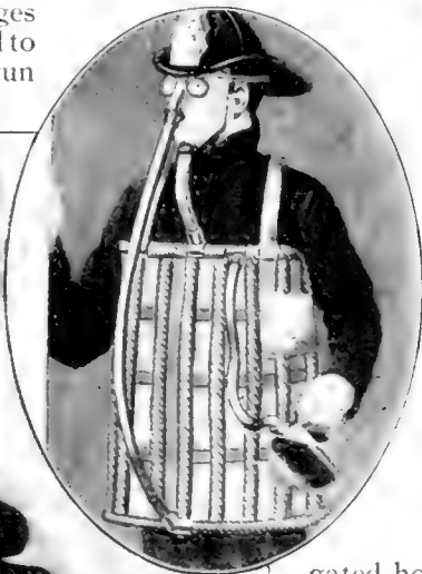
The gun is aimed by turning the head and fired by blowing through the tube in the mouth
